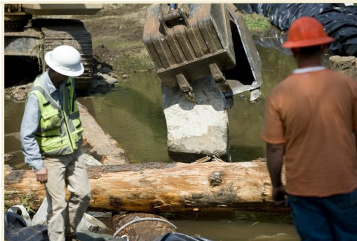
Above: Construction workers help a crane operator carefully place a boulder.
